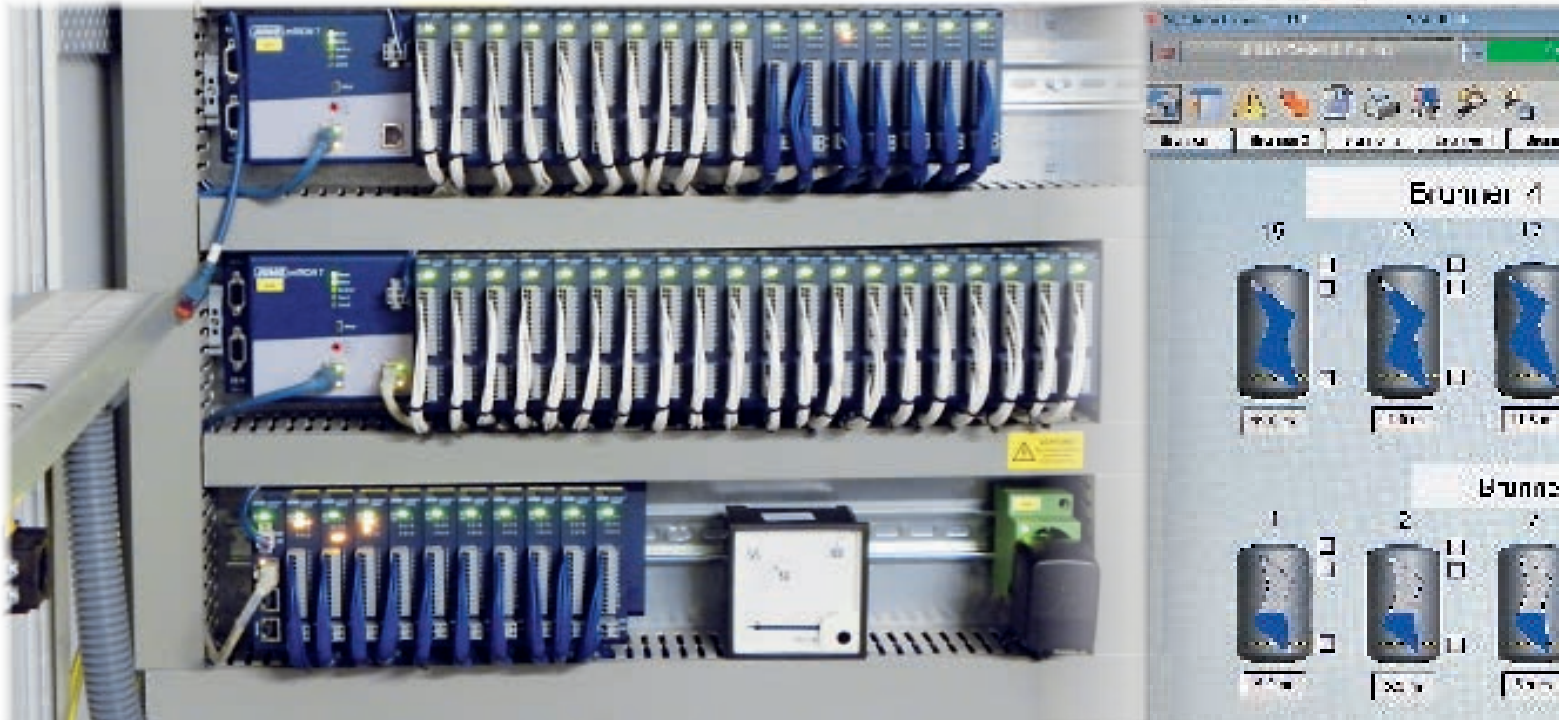
Fig. 1: Control cabinet with the JUMO mTRON T automation system
