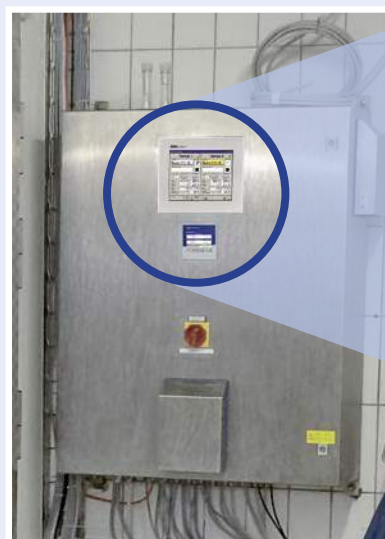
Ripening chamber with JUMO mTRON T panel and JUMO AQUIS touch P
