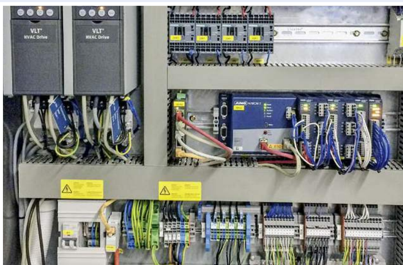
Installation situation of the JUMO mTRON T
