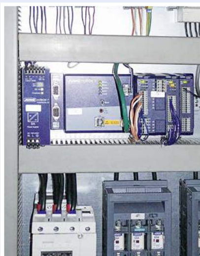
JUMO mTRON T in the control cabinet for temperature control in the tower furnace
