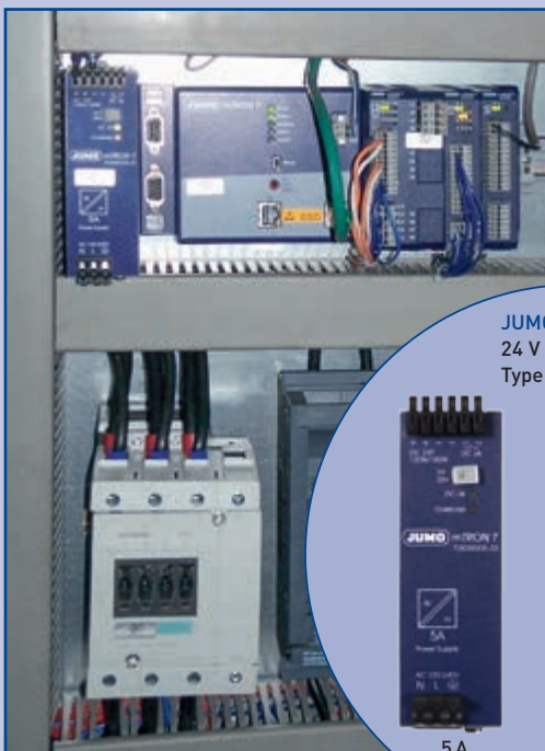
JUMO mTRON T in the control cabinet for temperature control in the tower furnace
