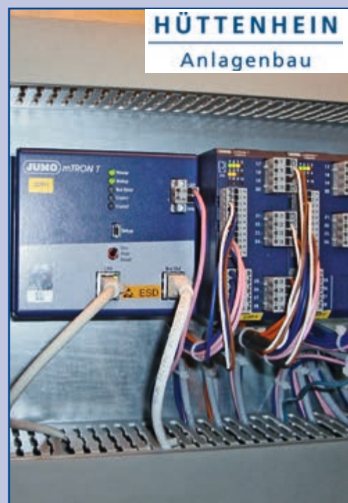
Installation situation of the JUMO mTRON T
